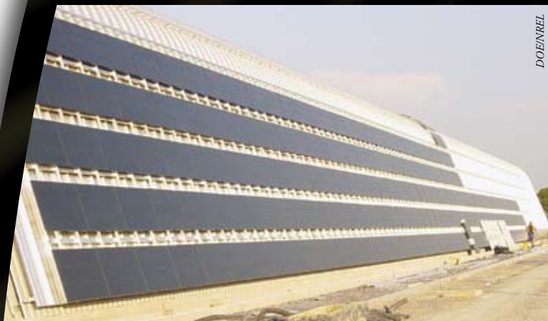
▲ An 84-kilowatt thin-film solar application on a building in Wales.
